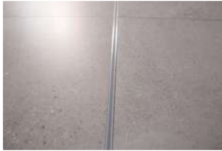
11- Take account of structural joints. Movement joints should be positioned as directed by the project designer. In general, do not design areas greater than 50-70 m 2 for interiors and half that for exteriors. Minimum joint width: 8 mm.
