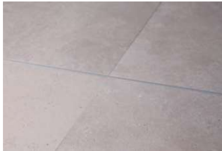
14- Joints should be grouted when the tiles are completely fixed to the substrate. In respect of paving, follow the recommendations of the adhesive manufacturer to ensure sufficient time is allowed before the floor is walked on or subjected to load. In this way movement and/or breakages are avoided.
